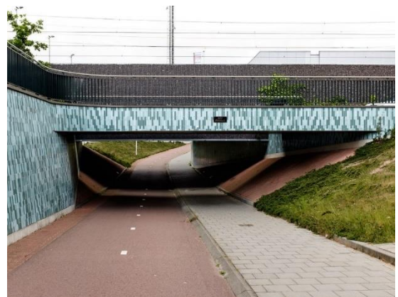
Underpass with bike path and foot path under railway in Den Dolder, NL
